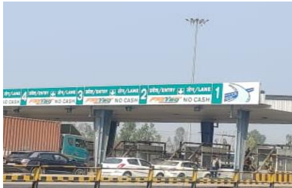
Chhappar Toll Plaza
