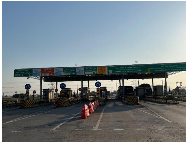
Odhaki Paipkhar Toll Plaza
