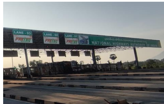
Marripalem Toll Plaza
