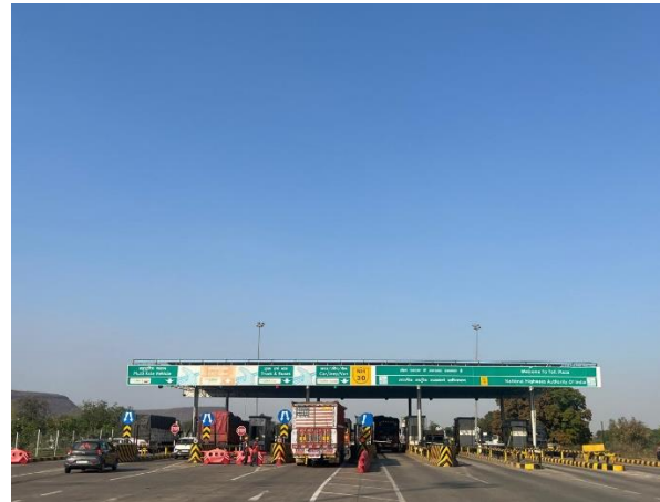
Kherwasani Toll Plaza
