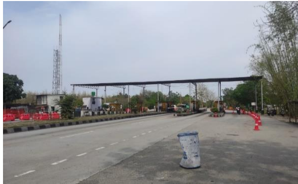
Patgaon Toll Plaza
